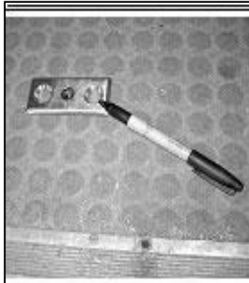
Figure 5 - Place each Floor Plate in place and mark the thru-bolt holes on each side
